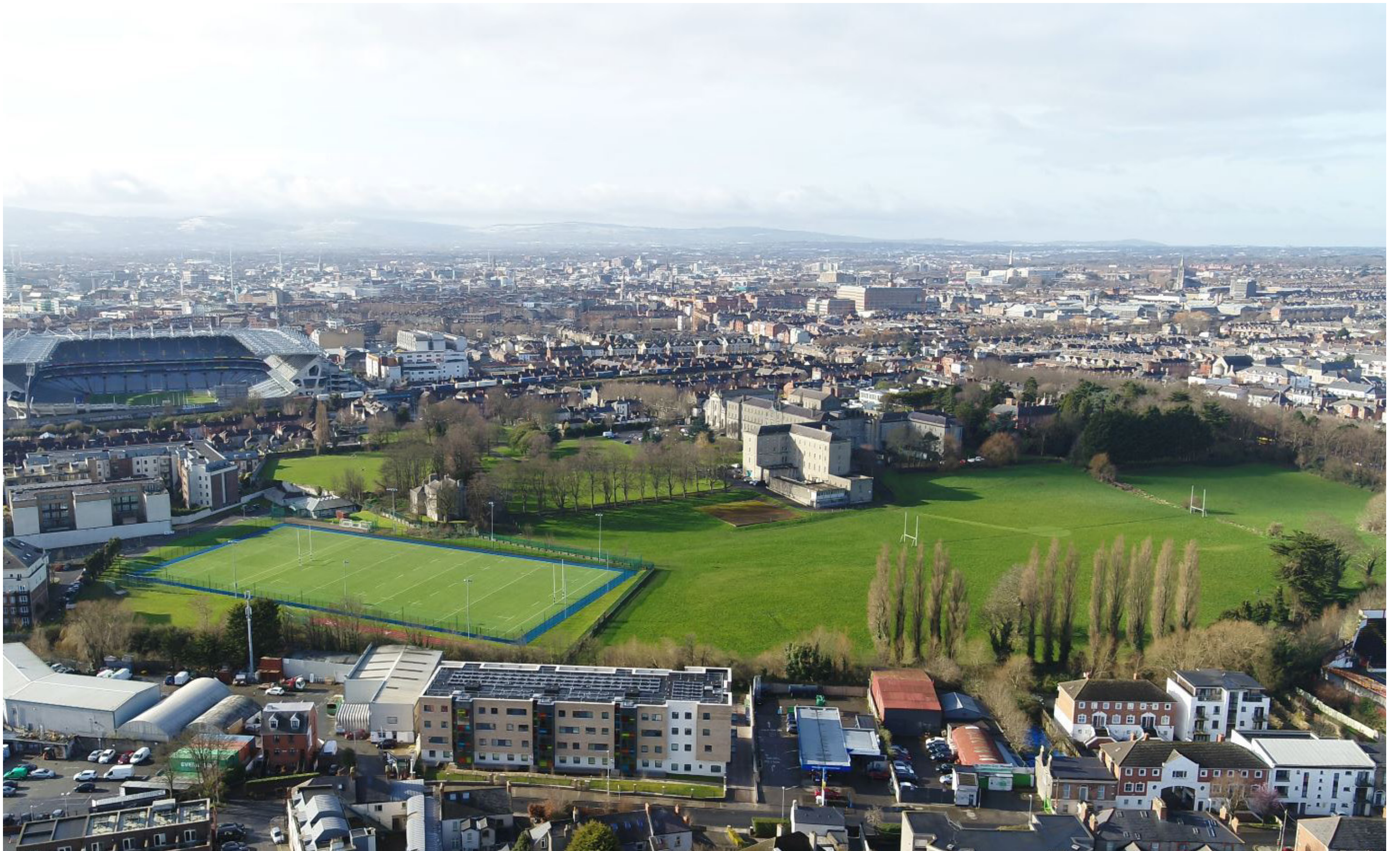
Aerial Photo - View Looking South
