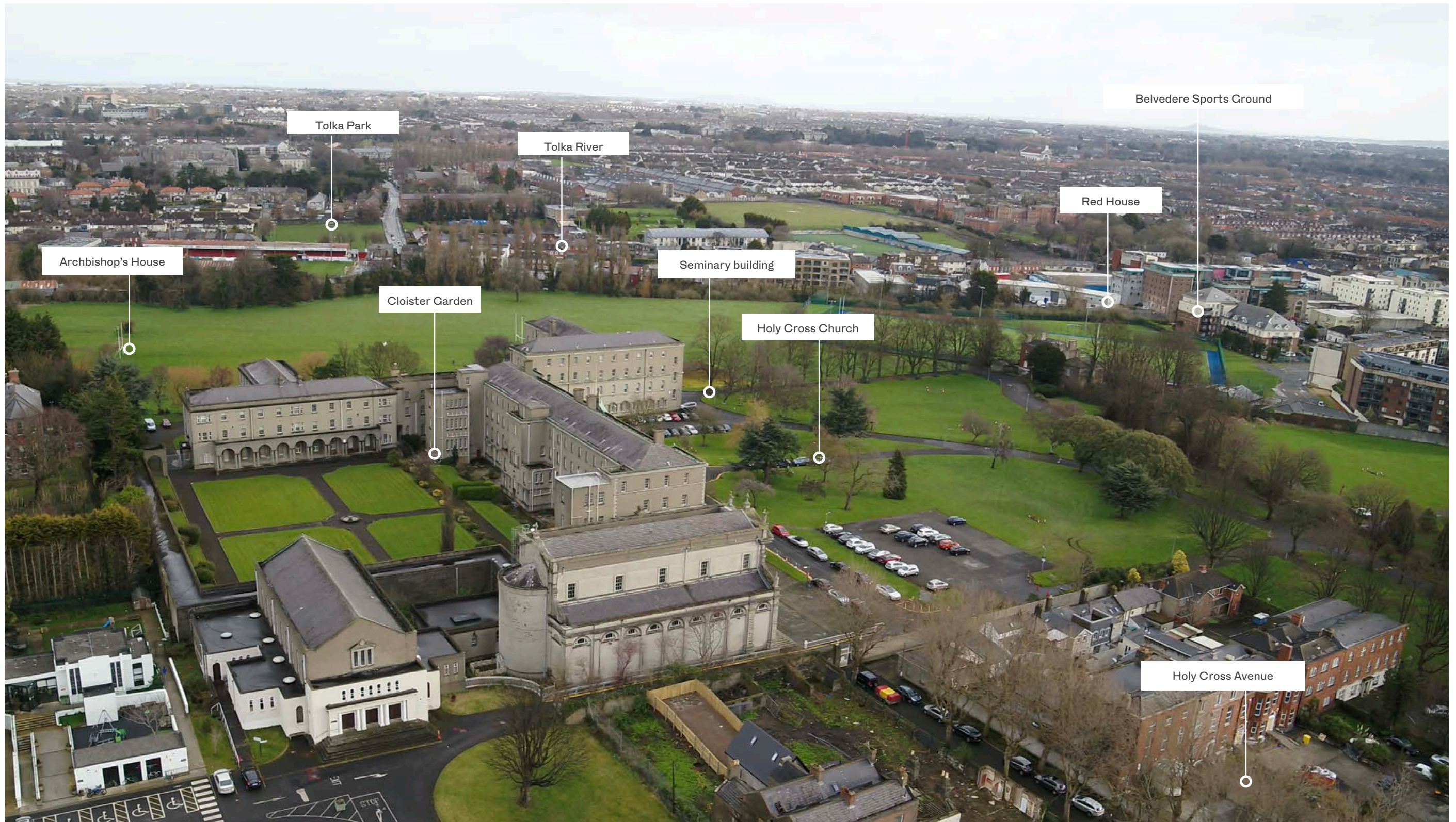
Aerial View - View from Clonliffe Road (Outside of site boundary) Looking North
